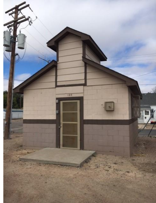
Figure 6: City of Yuma Wellhouse
